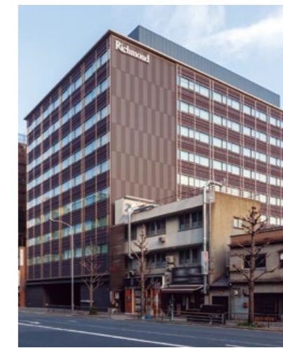
OVOL Kyoto Ekimae Building
