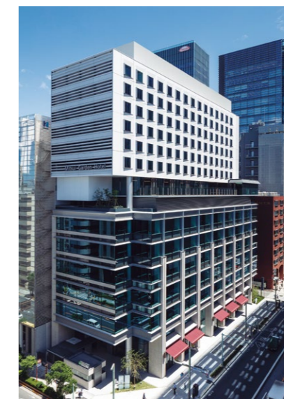
OVOL Nihonbashi Building
