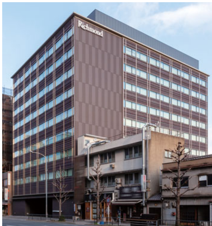
OVOL Kyoto Ekimae Building
