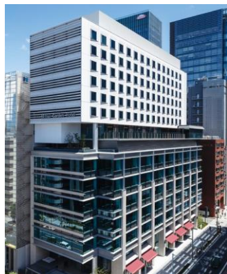
OVOL Nihonbashi Building
