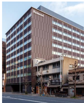
OVOL Kyoto Ekimae Building
